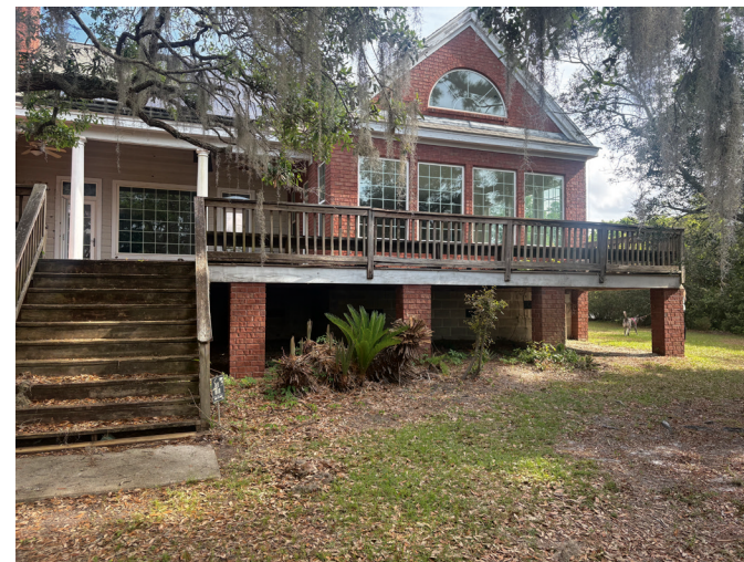
Before: 221 Lyman Hall Project
